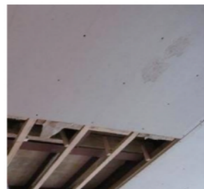
装饰拆除板产生垃圾
